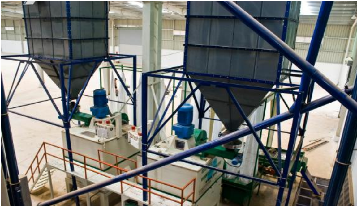
Photo: Nedcoffee Vietnam factory
