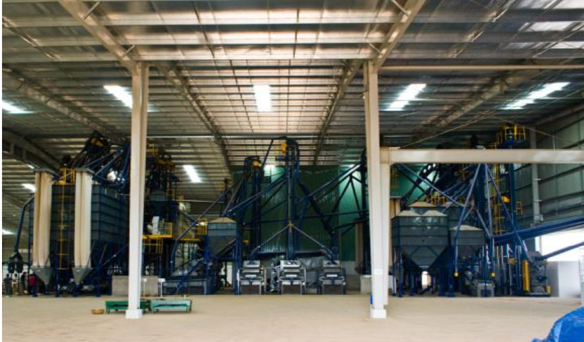
Photo: Nedcoffee Vietnam factory
